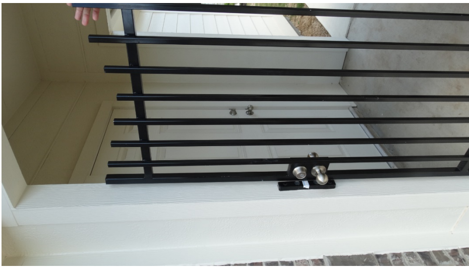
Entrance Gate — Deadbolt Lock
